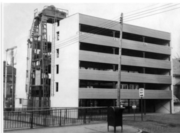
Crickelwood Apartments Garage. Steel has often been used in garage construction to reinforce concrete, but with coatings to protect against corrosion, it may also be used on its own. Photo by AISC Regional Engineer William L. Pascoli, PE.
