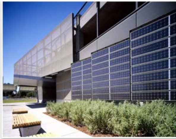
Fairfield Multimodal Transportation Center. This parking garage, designed by Stantec Architecture, uses photovoltaic cells and drought-tolerant landscaping, includes 400 parking stalls, bike lockers, telecommuting center, office building, 10 covered bus bays, electric vehicle charging ports, and plans for retail shops. Photo by David Wakely.
